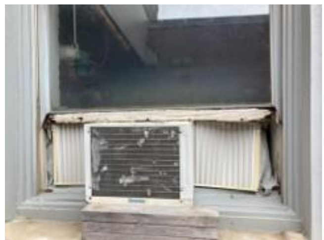
Central warehouse prior to HVAC upgrades.
